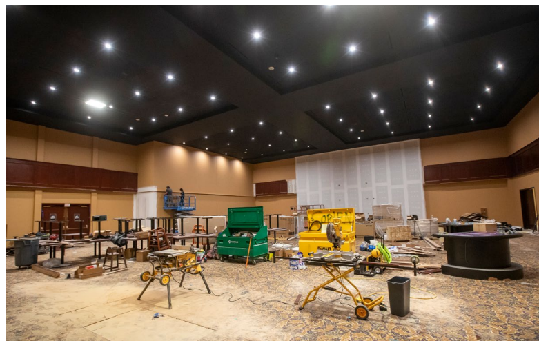
Construction of a new ballroom at the Grand Casino Hotel & Resort.
