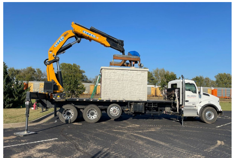
The new Rossville storm shelter being moved off the truck.
