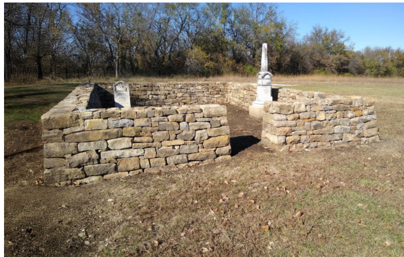
The Bourassa enclosure is pictured after being reconstructed in 2023.
